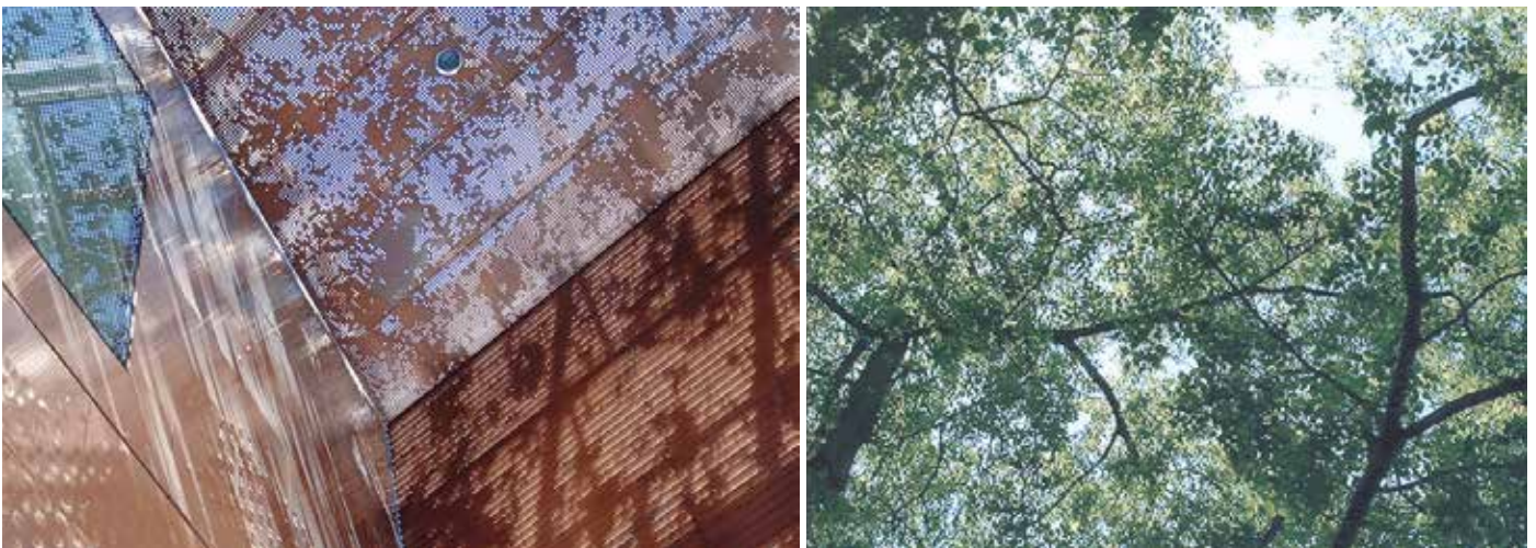
Figure 1. De Young Museum (Herzog & de Meuron) perforated copper panels and forest canopy effect.
